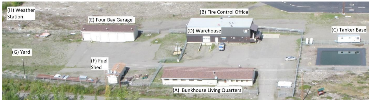
Figure 2. Aerial photo of the Dease Lake Fire Attack Base (FAB) facilities.
